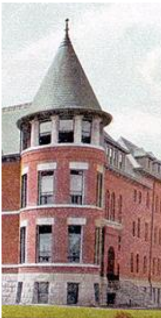
Originally the first infirmary rooms were located on the first floor, and then they were moved to the third and fourth floors. Notice fourth floor windows under roof. BVM Archives
