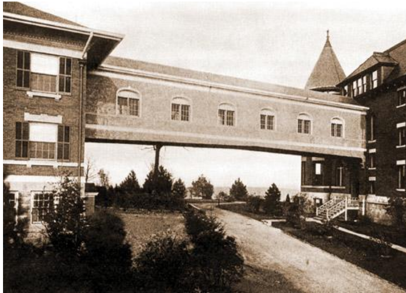
The bridge connected the motherhouse and the infirmary through a covered corridor over the drive-through outside the north entrance. It fit the needs of every weather or time for visits.
