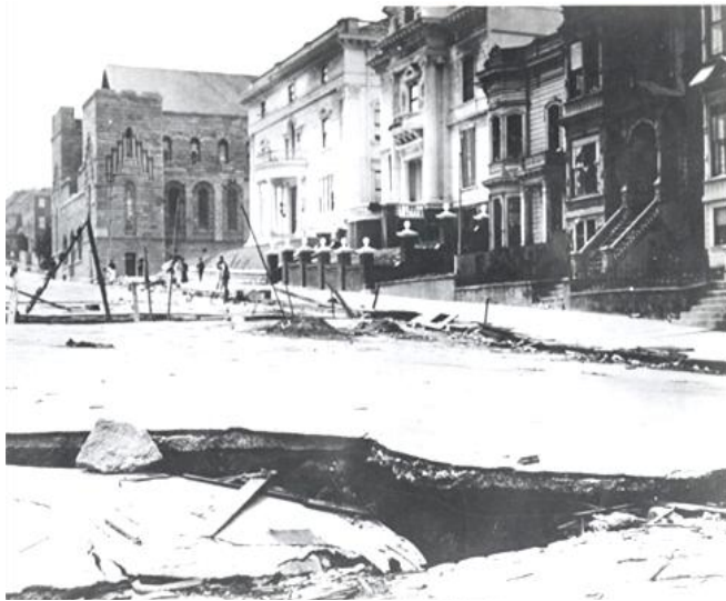
1906 Van Ness Avenue and St. Brigid Church after the earthquake San Francisco Public Library Photo Archives.
